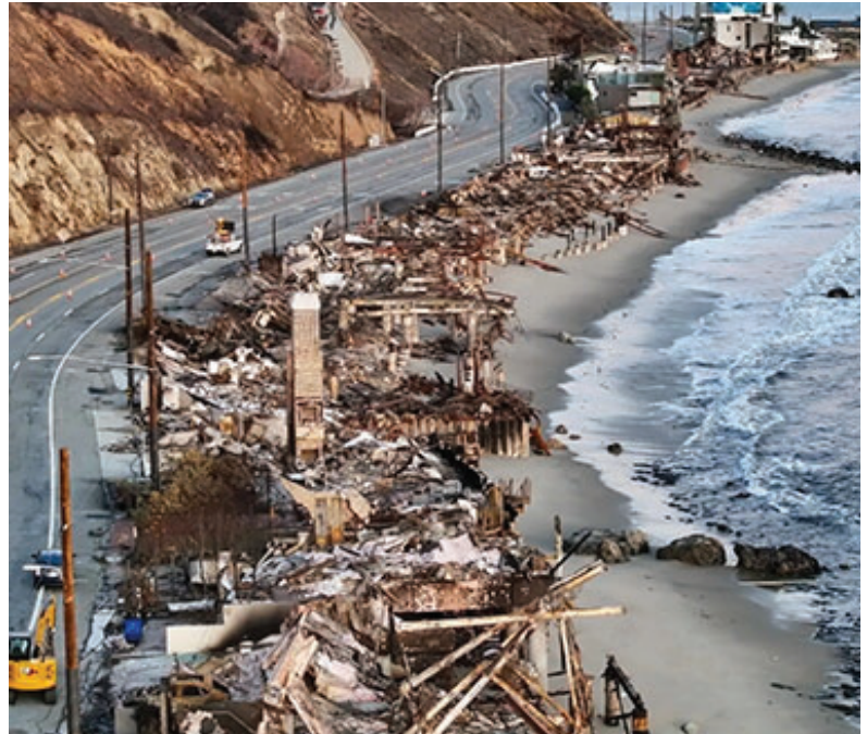
Wood poles wrapped with intumescent remain standing amid rubble left by the Palisades Fire. When disaster strikes, power must be restored before other restoration efforts can begin in earnest. Not having to install new poles accelerates the process.
