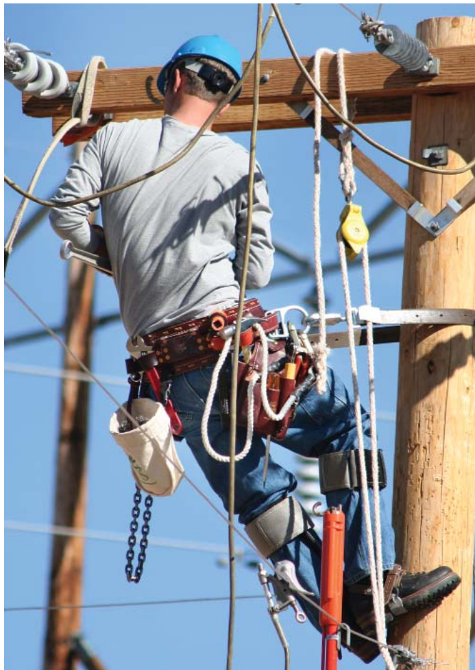
Figure 1 - Unlike underground systems, most repairs to electrical service can be done by linemen who have the appropriate gear to restore service quickly and economically.
