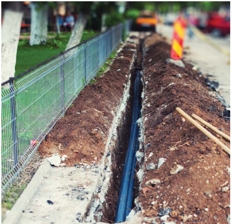
Figure 1 - Moving overhead lines underground is not only expensive, but creates significant disruptions in the areas where such work is done. Most undergrounding conversion projects require cutting through concrete or asphalt, forcing detours for traffic and pedestrians. Excavating also may be necessary to make repairs in underground systems should there be power failures.
