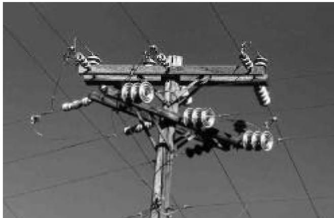
*Photo 7. Deadend structure with inadequate separation between jumper wires.*
