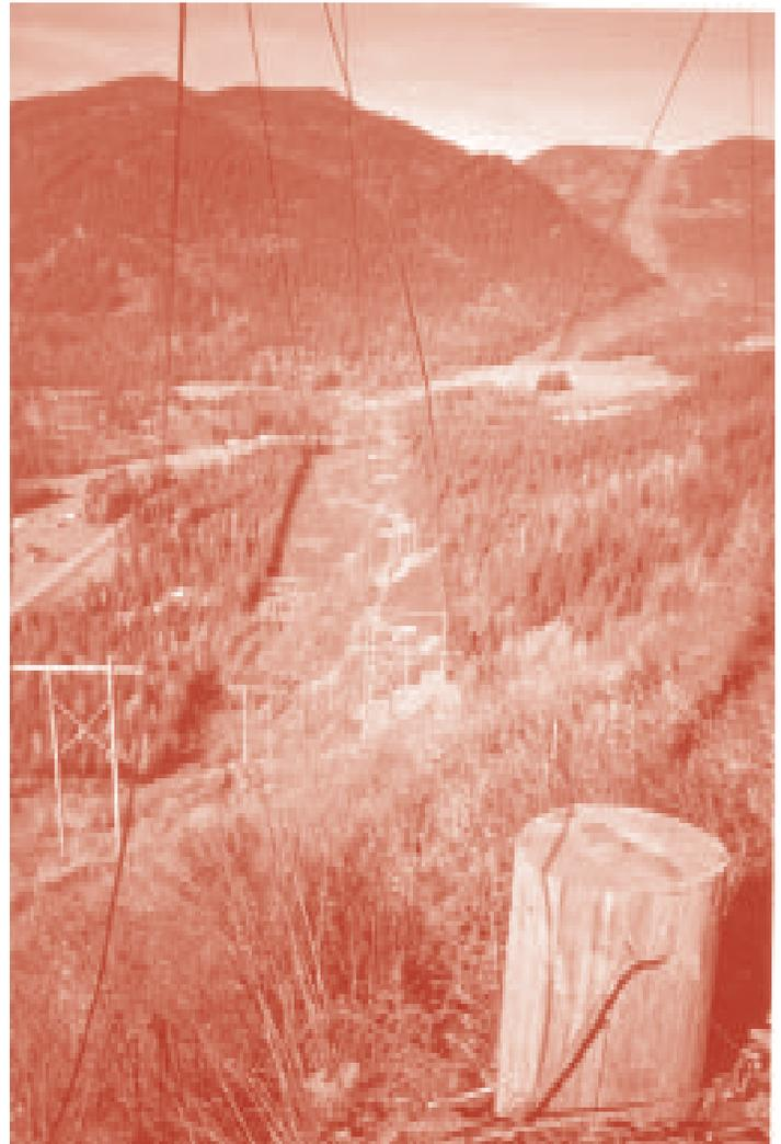
*To accommodate a narrow rugged right-of-way, a BC Hydro 230 KV circuit is relocated from an existing wood H-frame structure to a new double circuit H-frame structure.*
