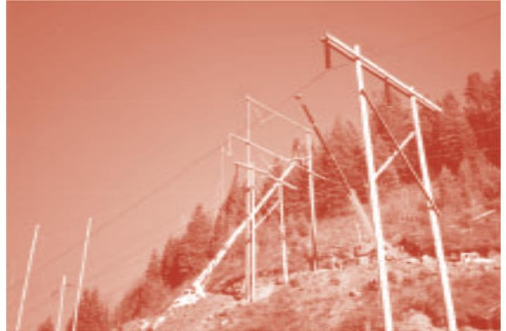
*An existing 230kV circuit is relocated from one of the wood H-frame lines to the new double circuit H-frame.*
