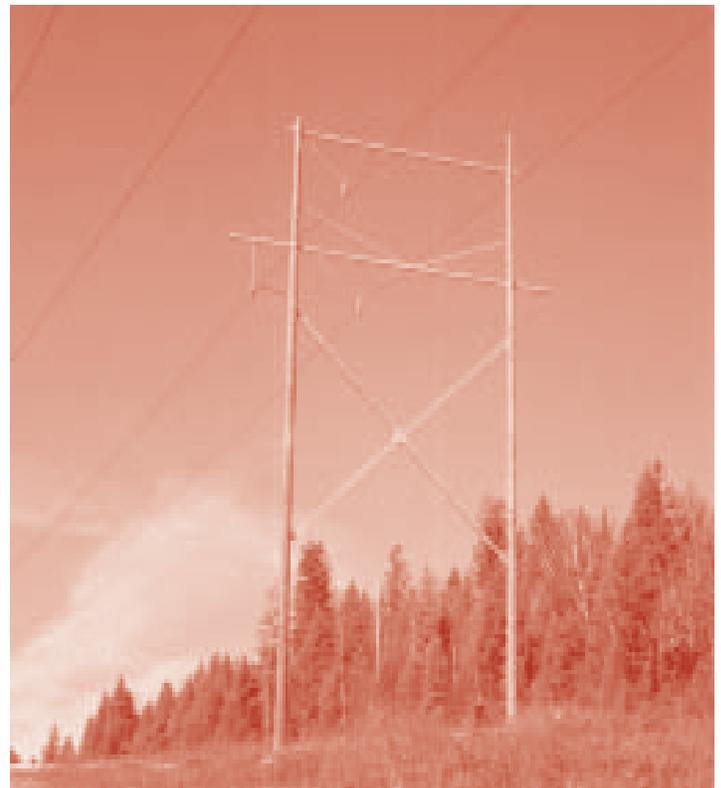
*125 ft. poles are shown here in the new double circuit wood H-frame structure. The relocated circuit is on the left and the new Columbia Power Circuit will be installed on the right side of the structure in Spring 2001.*
