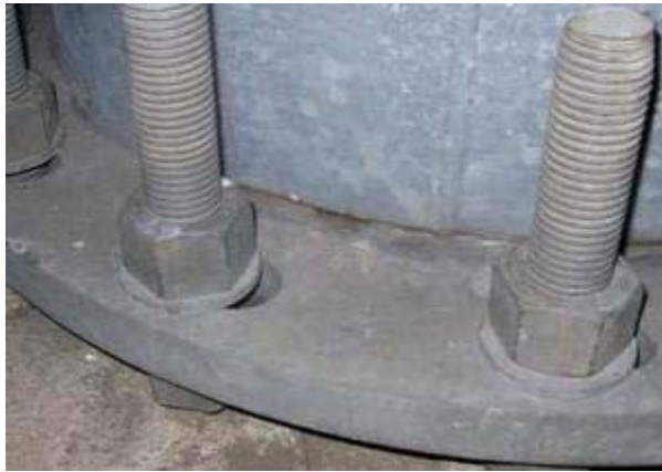
Base plate of stadium light pole
